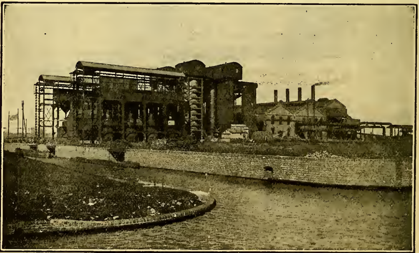
FIG. 264.—Mond Byproduct Gas Plant, at Dudley Port, South Staffordshire, England.
